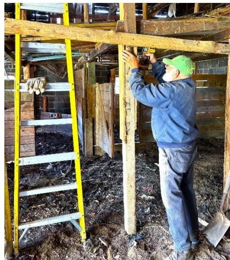
Ed Williamson reinforcing the DART storage barn on clean-up day, 12/7/24
